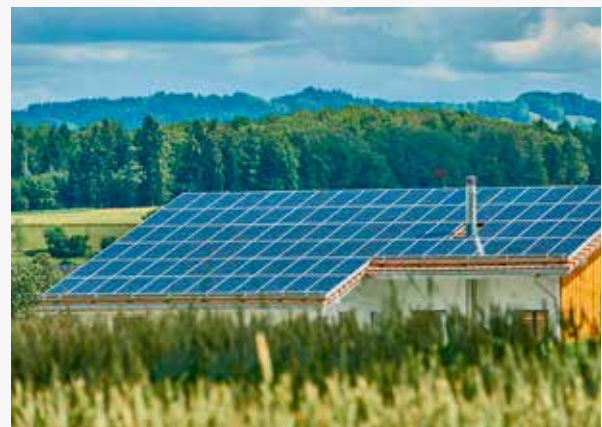
Photo: SolarX installation.
