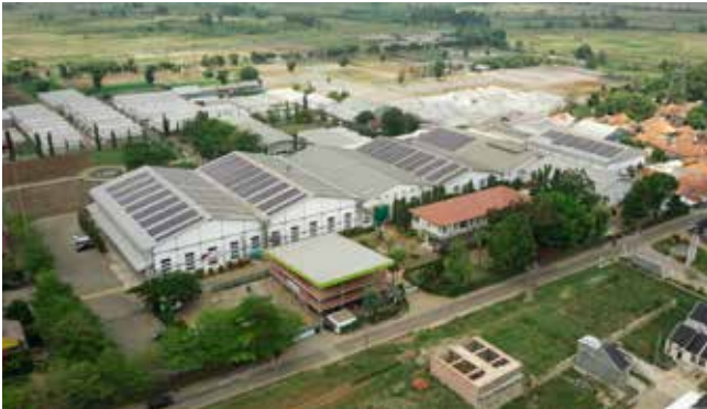
Indonesia: solar rooftop installation. © Xurya Daya Indonesia.
