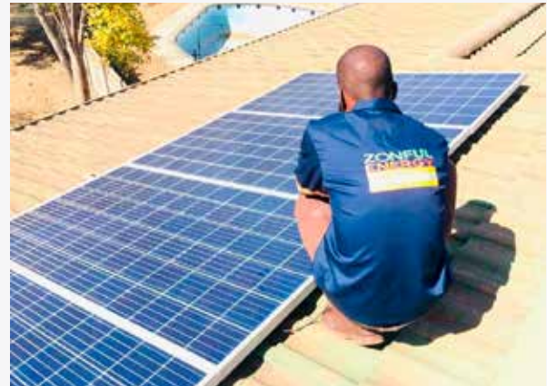
Photo: Zonful; solar panel installation.
