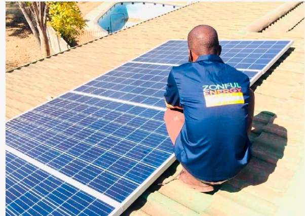
Photo: Zonful; solar panel installation.
