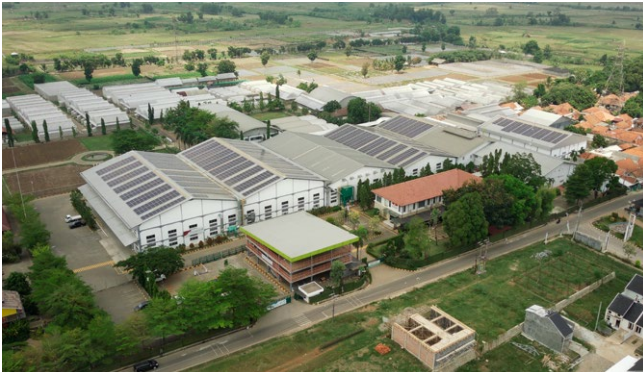
Indonesia: solar rooftop installation. © Xurya Daya Indonesia.
